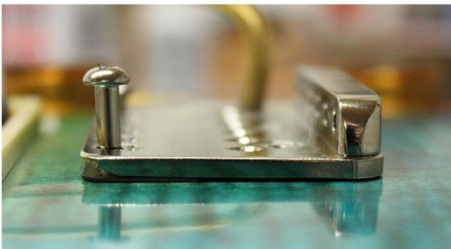
Screw the bearing screw (which will be under the sixth string) down until the screw head touches the plate and then as you screw down a little more you will see the back edge of the plate lift. Bring the screw down until the plate is just sat nicely flat on the shim. In this position the angle between the vertical of the bearing screws and the top of the plate should be at 90 degrees as per the pic below and this is the correct height setting.
